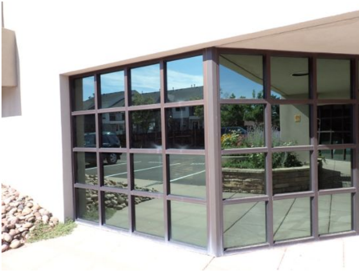
The majority of the exterior envelope of the structure appeared to be in fair condition at the time of the inspection.
