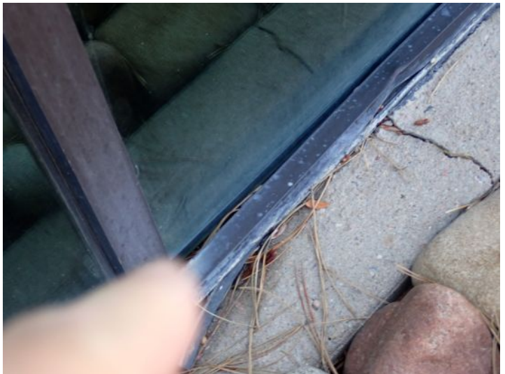
The concrete perimeter beam located on the lower west side of the structure had failed and was settling toward the structure at the time of the inspection. Recommend repairs by a licensed contractor.
