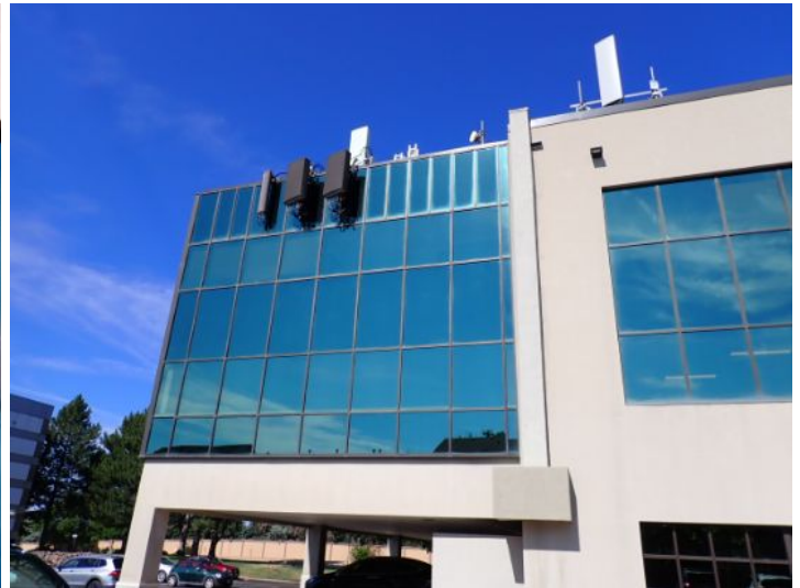
The majority of the exterior envelope of the structure appeared to be in fair condition at the time of the inspection.
