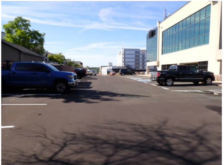
The parking lot surface was in fair condition at the time of the inspection.
