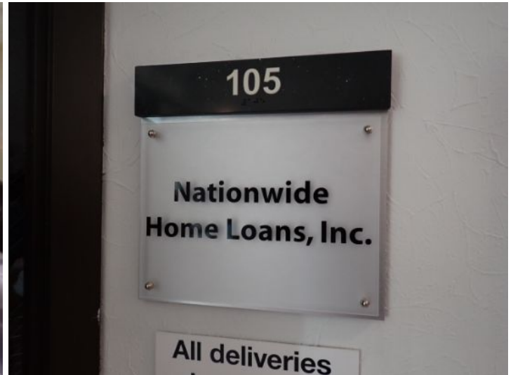
The majority of the interiors of the office suites appeared to be in fair condition at the time of the inspection.
