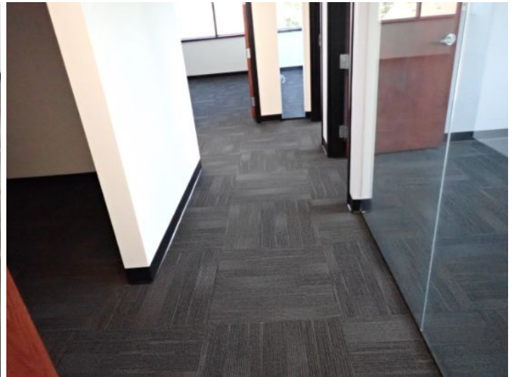
The majority of the interiors of the office suites appeared to be in fair condition at the time of the inspection.
