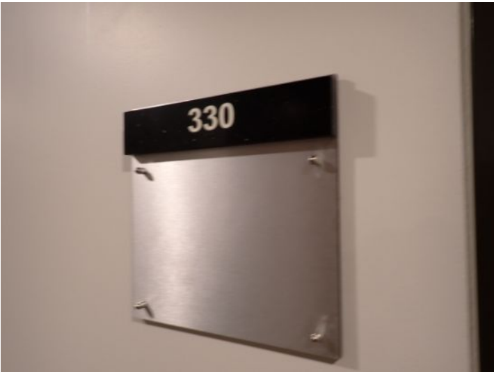
Suite 330: Significant moisture damage noted in the cabinet floor below break area sink. No GFCI protection noted near sink. VCT flooring damage noted. Recommend repairs.
