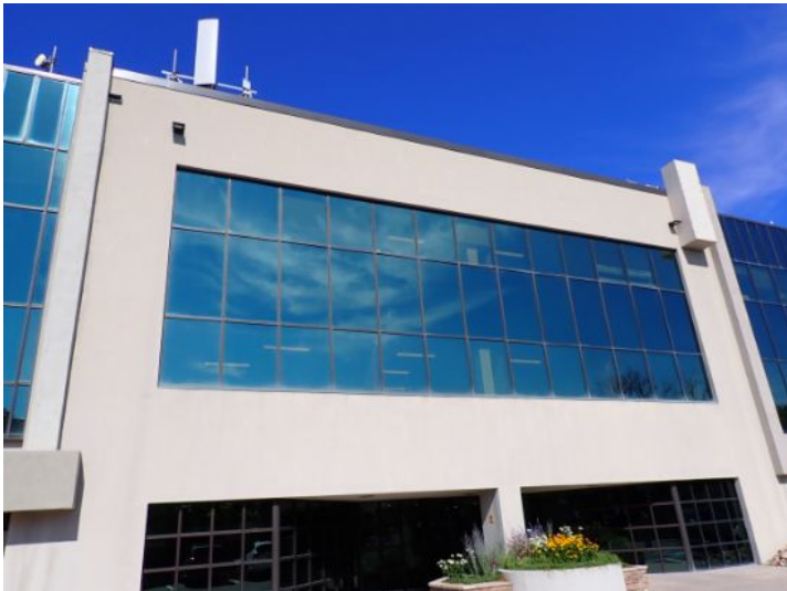
The majority of the exterior envelope of the structure appeared to be in fair condition at the time of the inspection.
