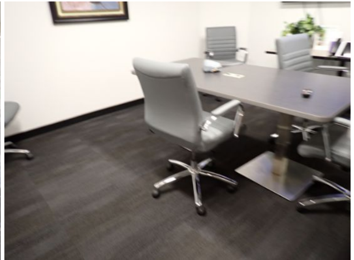
The majority of the interiors of the office suites appeared to be in fair condition at the time of the inspection.
