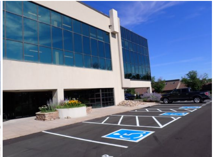
The majority of the exterior envelope of the structure appeared to be in fair condition at the time of the inspection.
