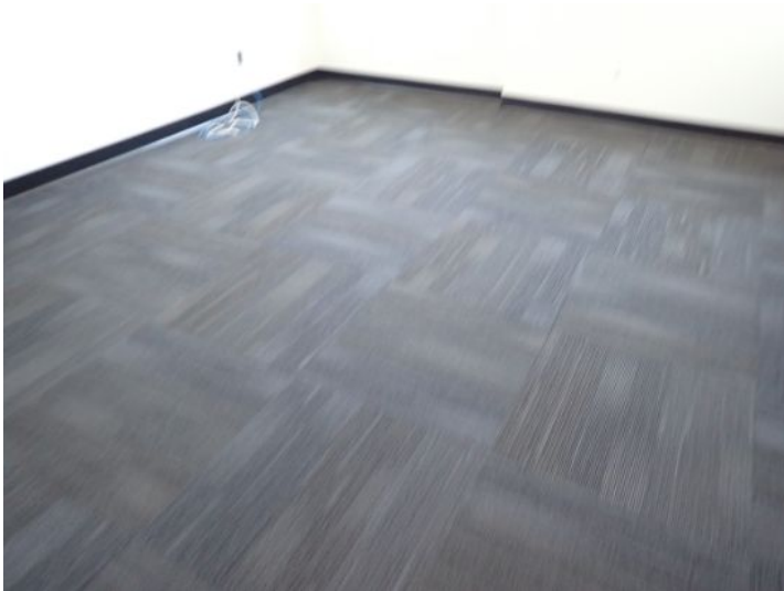
The majority of the interiors of the office suites appeared to be in fair condition at the time of the inspection.
