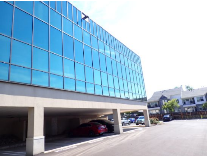
The majority of the exterior envelope of the structure appeared to be in fair condition at the time of the inspection.
