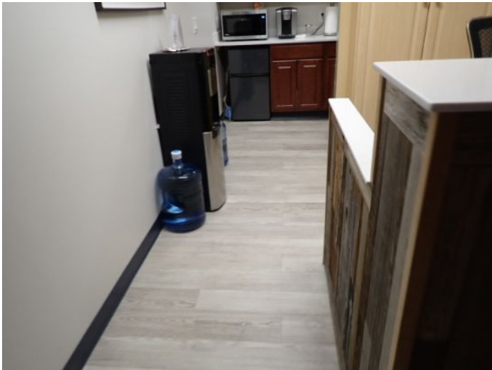
The majority of the interiors of the office suites appeared to be in fair condition at the time of the inspection.
