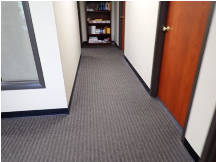
The majority of the interiors of the office suites appeared to be in fair condition at the time of the inspection.
