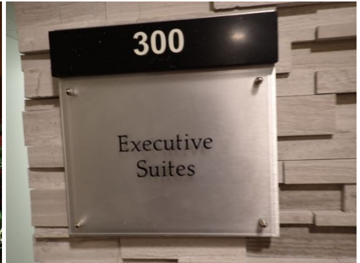
The majority of the interiors of the office suites appeared to be in fair condition at the time of the inspection.
