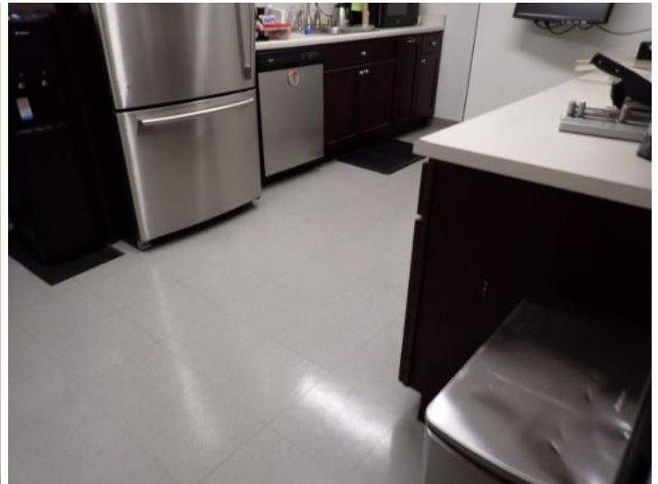
The majority of the interiors of the office suites appeared to be in fair condition at the time of the inspection.
