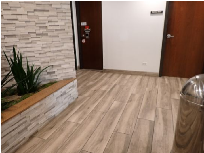
The majority of the common areas appeared to be in fair condition at the time of the inspection.
