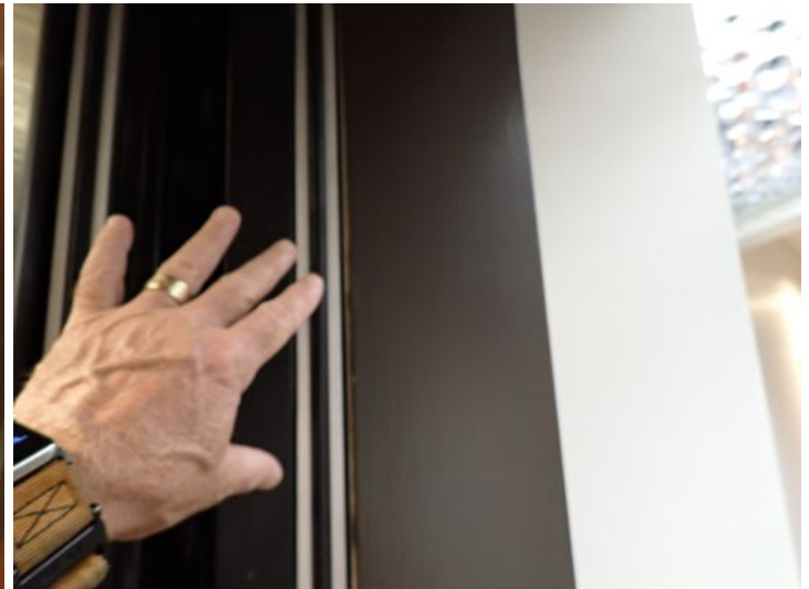
No floor markings noted on the individual floors at the elevator exit. Recommend repairs by a licensed contractor.
