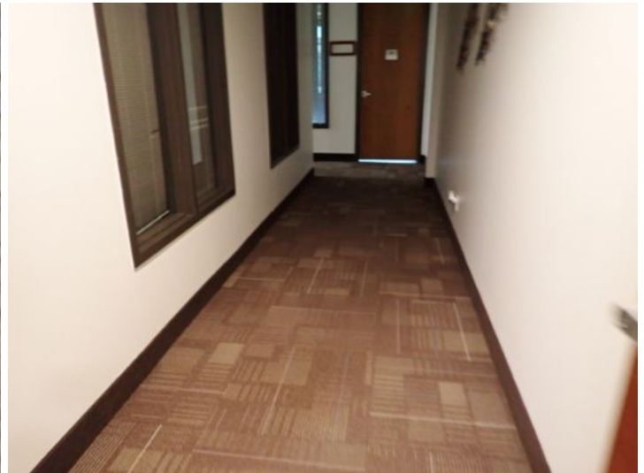
The majority of the interiors of the office suites appeared to be in fair condition at the time of the inspection.
