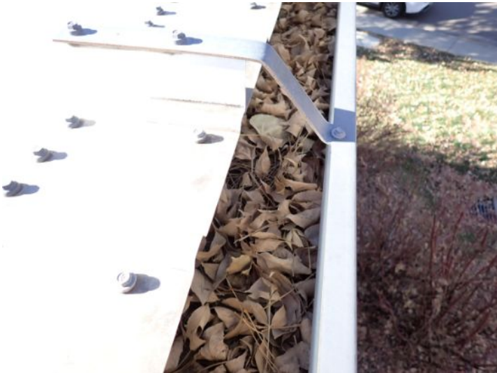
Roof gutter systems were clogged with debris at the time of the inspection. Recommend repairs by a licensed contractor.
