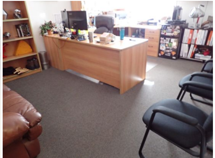
The majority of the interior of the office area appeared to be in fair condition at the time of the inspection.
