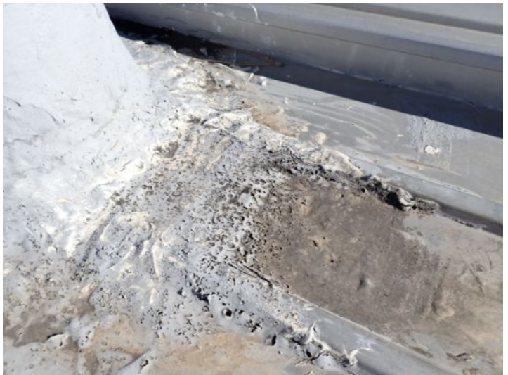
The sealant around the roof penetrations appeared to have reached its serviceable life expectancy and may begin leaking soon. Recommend repairs as needed by a licensed contractor.
