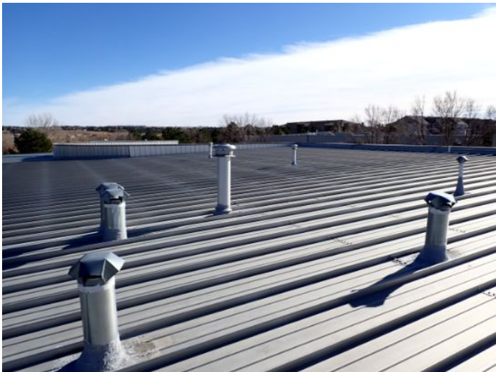
The majority of the standing seam metal roofing system appeared to be in fair condition at the time of the inspection.
