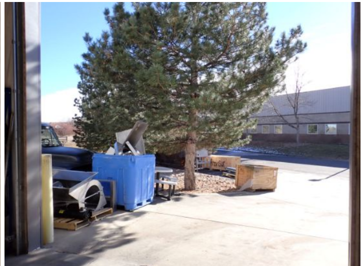
The overhead doors and personnel doors were tested and functional at the time of the inspection.
