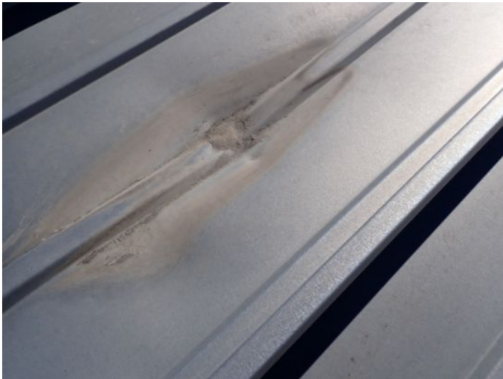
There were a couple of areas noted on the roof top where there were fairly large indentation's noted in the steel roofing system causing ponding. Recommend repairs by a licensed contractor.
