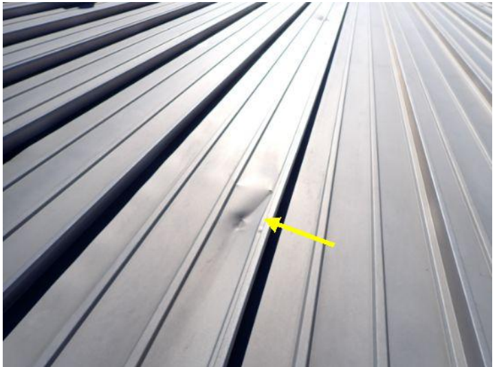
There were a couple of areas noted on the roof top where there were fairly large indentation's noted in the steel roofing system causing ponding. Recommend repairs by a licensed contractor.
