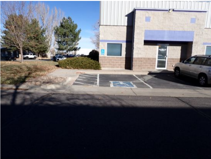
ADA parking was clearly marked at the time of the inspection.
