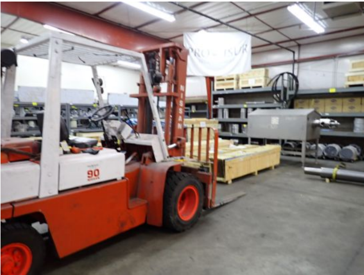
The majority of the interior of the warehouse area appeared to be in fair condition at the time of the inspection.
