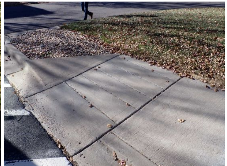
The ADA ramps were checked for proper grade and no significant issues were noted at the time of the inspection.
