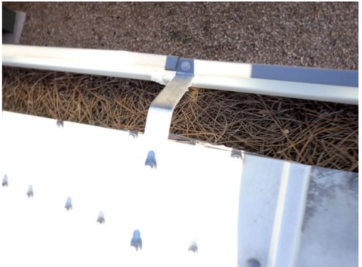
Roof gutter systems were clogged with debris at the time of the inspection. Recommend repairs by a licensed contractor.
