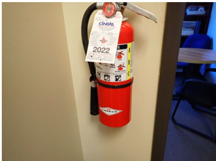
There were fire extinguishers located within the structure
