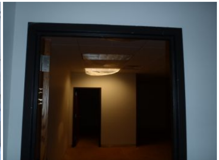
At the time of the inspection there was one overhead light that remained on in each office after all switches were turned off. Recommend evaluation by a licensed electrical contractor when they come in to run the new electrical.
