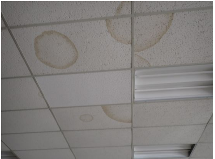
Unit 108-107: Vacant: Unit will require significant renovations prior to installing tenant. Active moisture noted in interior wall with possible microbial growth. Significant drywall damage noted in ceiling in loading dock area. Basement area in poor condition. Basement bathrooms in poor condition. Electrical not working at the time of the inspection. Moisture intrusion/damage noted in basement walls. Recommend repairs as needed by a licensed contractor.
