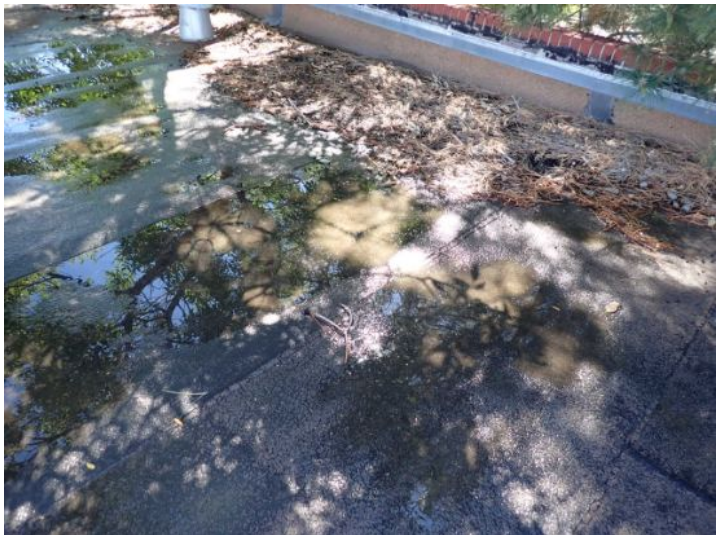
The rolled asphalt composition roofing system located above the south end of the west wing was in poor condition with excessive ponding, deferred maintenance, excessive debris and excessive granular loss at the time of the inspection. Recommend complete replacement by licensed roofing contractor.
