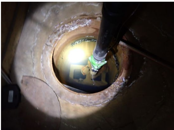
Sump pits and pump systems not functional in the basement below units 108-107 at the time of the inspection. Recommend repairs by a licensed contractor.
