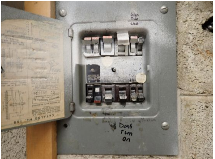
Old Federal Pacific Stab Lock breaker systems noted in some of the units at the time of the inspection. These systems have been proven to be safety/fire issues. Recommend replacement of all FPE panels and stab lock breaker systems by a licensed contractor prior to taking possession of the property.
