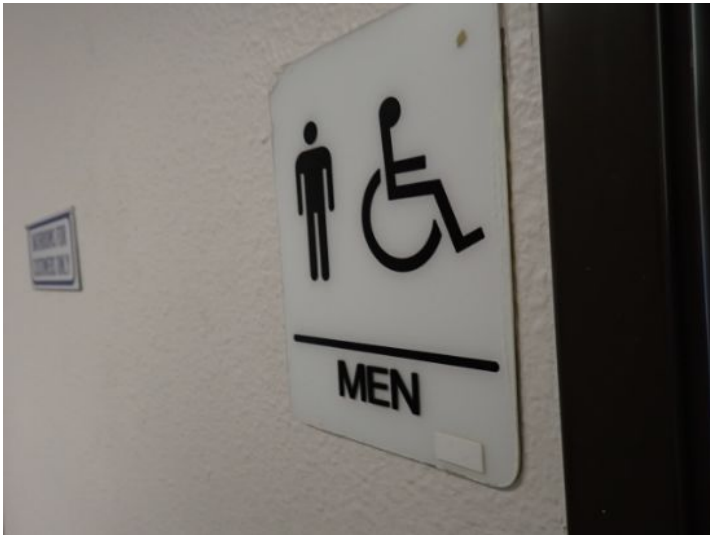
The common area restrooms in the office building and mall areas were tested and functional at the time of the inspection.
