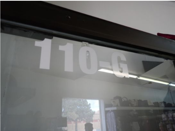
Unit 110G: Acoustical tile ceiling damage noted. Missing knockouts noted in electrical panel. Recommend repairs.
