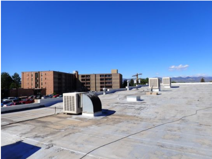
The rolled torch down roofing system above what used to be the old theater it is now currently being used as the office area appeared to be original to the structure and was showing signs of hail damage excessive ponding where and patching. Recommend replacement by licensed contractor.
