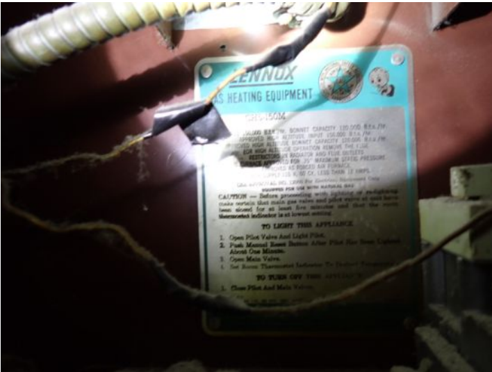
There was an old gas fired forced air furnace located in the main level of the old theater building that although functional had far surpassed its serviceable life expectancy and could be considered a safety/health hazard. Recommend replacement by a licensed contractor.
