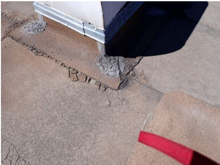
The rolled asphalt composition roofing system located above the south end of the west wing was in poor condition with excessive ponding, deferred maintenance, excessive debris and excessive granular loss at the time of the inspection. Recommend complete replacement by licensed roofing contractor.
