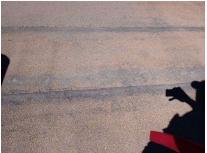
The rolled asphalt composition roofing system located above the south end of the west wing was in poor condition with excessive ponding, deferred maintenance, excessive debris and excessive granular loss at the time of the inspection. Recommend complete replacement by licensed roofing contractor.
