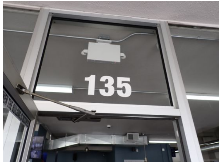
Unit 135: No significant findings noted at the time of the inspection.
