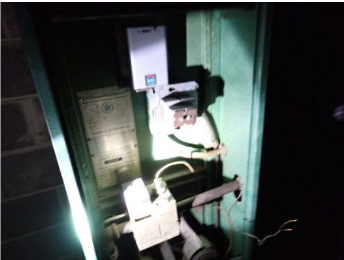
Old gas fired furnace for the basement area of units 108-107 was in poor condition and requires complete replacement.
