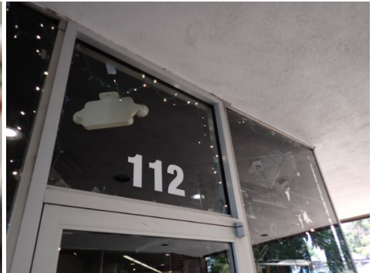
Unit 112: No significant findings noted at the time of the inspection.
