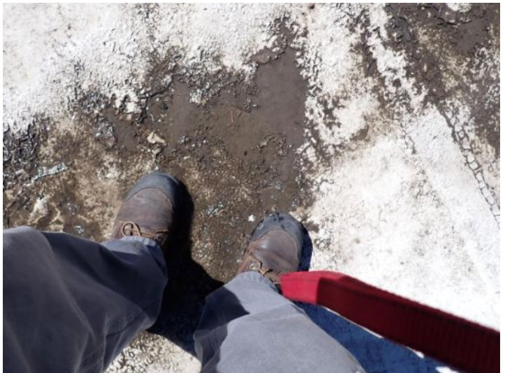
The rolled torch down roofing system above what appeared to be the old family dollar store and the vacant unit was an extremely poor condition excessive ponding feeling coding possible hail damage and excessive wear noted at the time of the inspection. Recommend complete replacement by licensed contractor.
