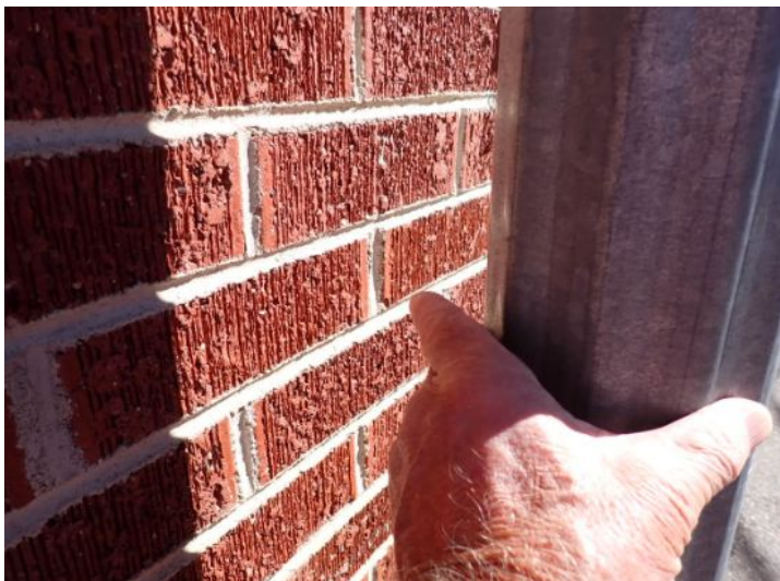
Loose down spouts. Recommend repairs.
