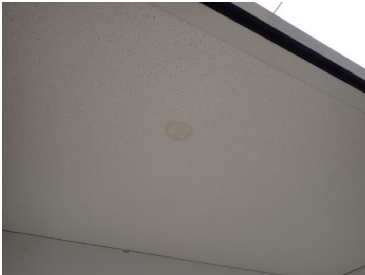
Unit 104: Sub standard plumbing noted below vanity sink. Past moisture staining noted in ceiling. Recommend repairs.
