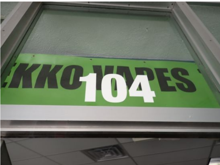
Unit 104: Sub standard plumbing noted below vanity sink. Past moisture staining noted in ceiling. Recommend repairs.
