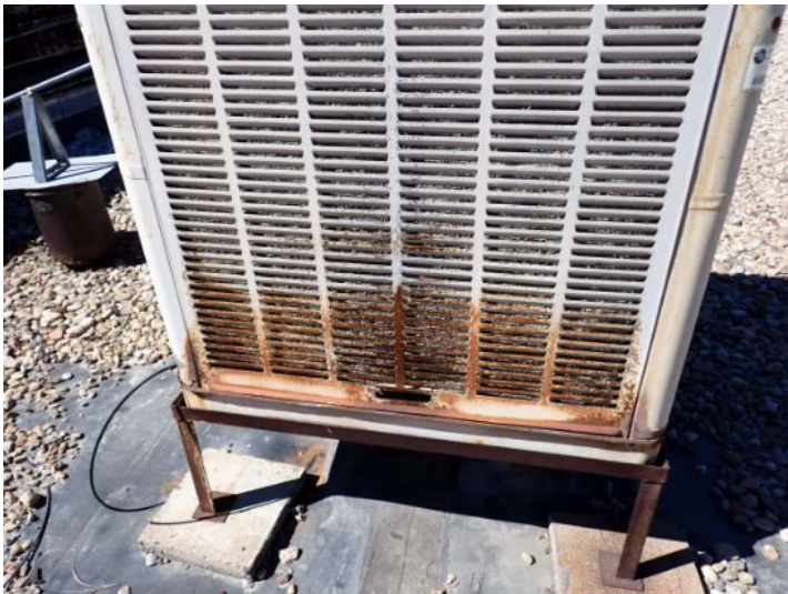
The swamp coolers for units 108-107 were in poor condition at the time of the inspection. Unit will require new heating/cooling systems for new tenant. Recommend repairs by a licensed contractor.
