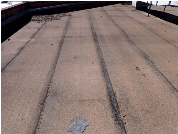
The rolled asphalt composition roofing system located above the south end of the west wing was in poor condition with excessive ponding, deferred maintenance, excessive debris and excessive granular loss at the time of the inspection. Recommend complete replacement by licensed roofing contractor.
