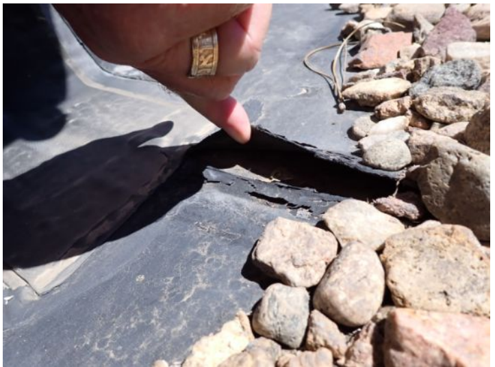
The gravel coated EPDM roofing membrane located towards the north end of the west structure was showing signs of significant ponding and deferred maintenance at the time of the inspection. Recommend repair by licensed contractor.
