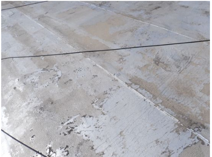
The rolled torch down roofing system above what used to be the old theater it is now currently being used as the office area appeared to be original to the structure and was showing signs of hail damage excessive ponding where and patching. Recommend replacement by licensed contractor.
