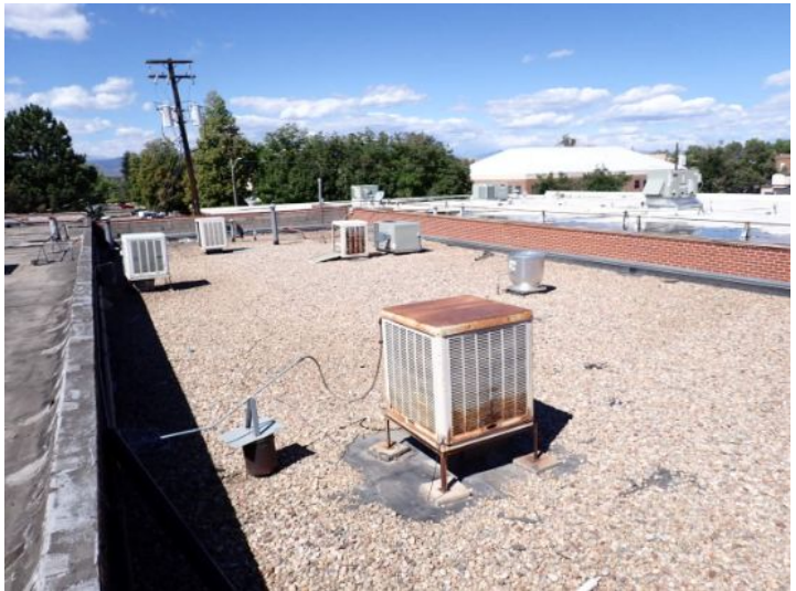
The swamp coolers for units 108-107 were in poor condition at the time of the inspection. Unit will require new heating/cooling systems for new tenant. Recommend repairs by a licensed contractor.
