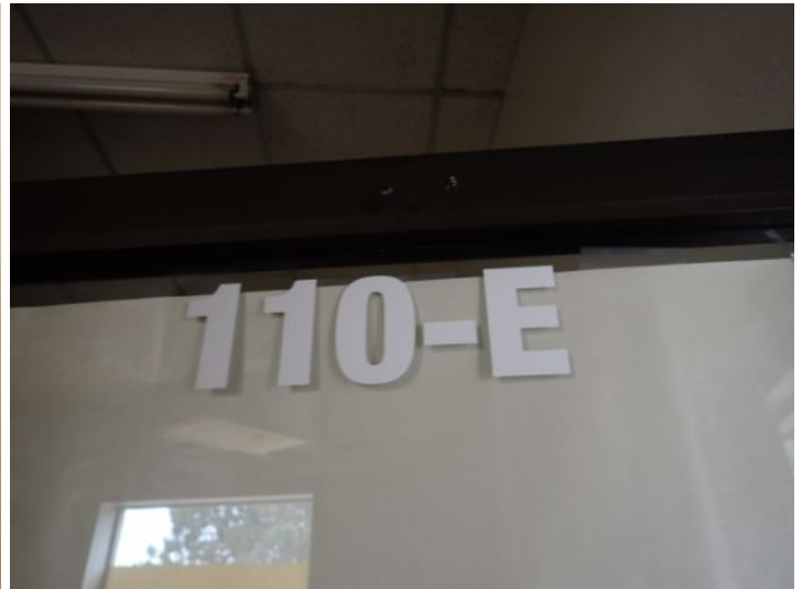
Unit 110E: Unit was vacant and will require renovations prior to placing a tenant. Recommend repairs by a licensed contractor.
