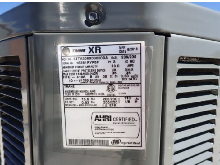
CU 5: Trane: M/N 4TTA3060D3000DA S/N 18351RYP5F. Manufacture year 2018.
