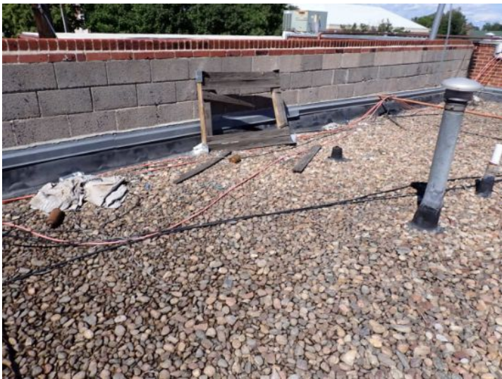
The gravel coated EPDM roofing membrane located towards the north end of the west structure was showing signs of significant ponding and deferred maintenance at the time of the inspection. Recommend repair by licensed contractor.
