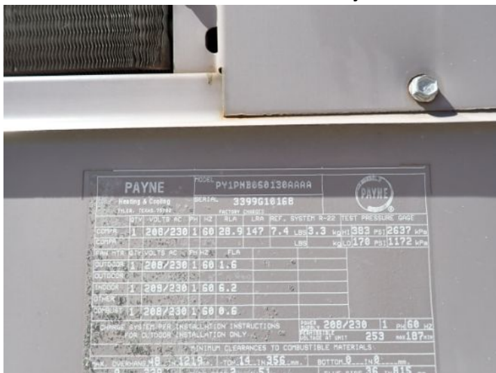
RTU 32: Payne: M/N PY1PNB060130AAAA S/N 3399G10168. Manufacture year 1999.
