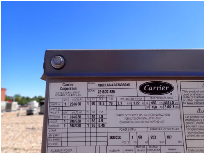
RTU 28: Carrier: M/N 48KCEA04A2A3A0A0A0 S/N 2318C51885. Manufacture year 2018.
