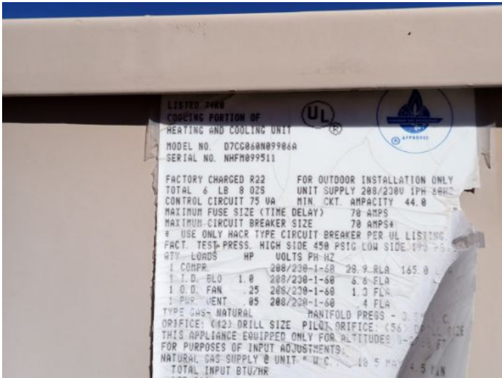
RTU 8: York: M/N D7CG060N09906A S/N NHFM099511. Manufacture year 1997.
