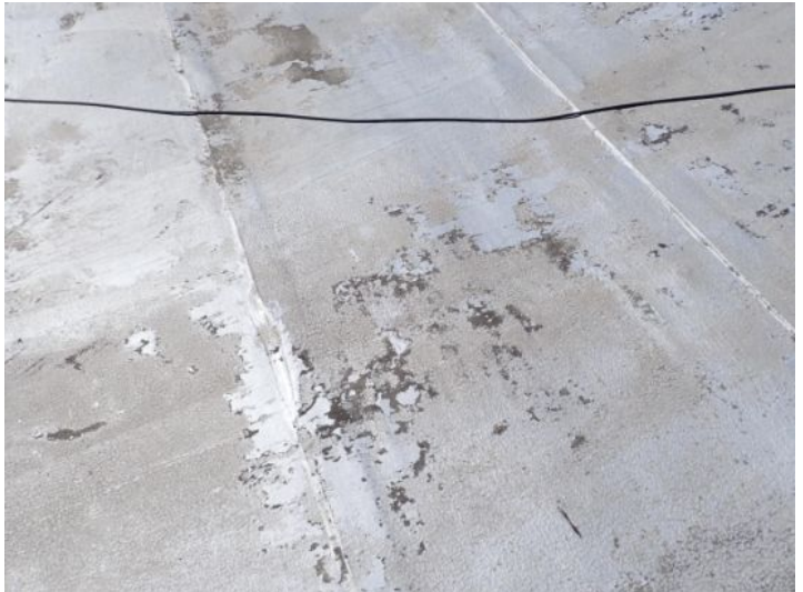
The rolled torch down roofing system above what used to be the old theater it is now currently being used as the office area appeared to be original to the structure and was showing signs of hail damage excessive ponding where and patching. Recommend replacement by licensed contractor.
