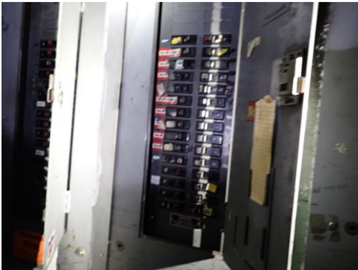
The nominal serviceable life expectancy of an electrical breaker system is 30 years. Based on the inspectors findings at the time of the inspection there were multiple panels and breaker systems that appeared to have surpassed their serviceable life expectancy. Recommend repair/replacement of these systems by a licensed electrician prior to taking possession of the property.
