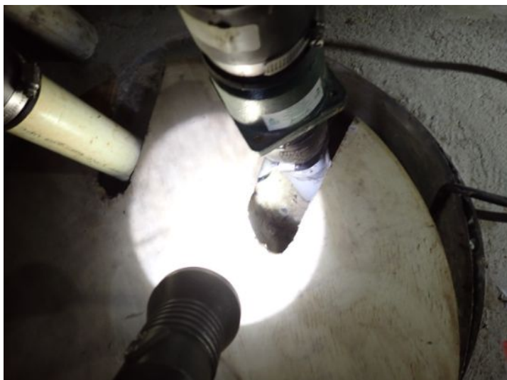
Sump pits and pump systems not functional in the basement below units 108-107 at the time of the inspection. Recommend repairs by a licensed contractor.
