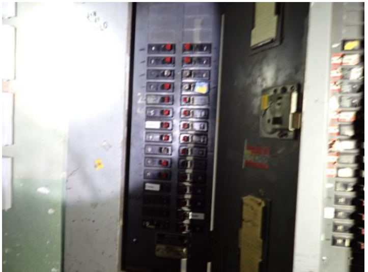
The nominal serviceable life expectancy of an electrical breaker system is 30 years. Based on the inspectors findings at the time of the inspection there were multiple panels and breaker systems that appeared to have surpassed their serviceable life expectancy. Recommend repair/replacement of these systems by a licensed electrician prior to taking possession of the property.
