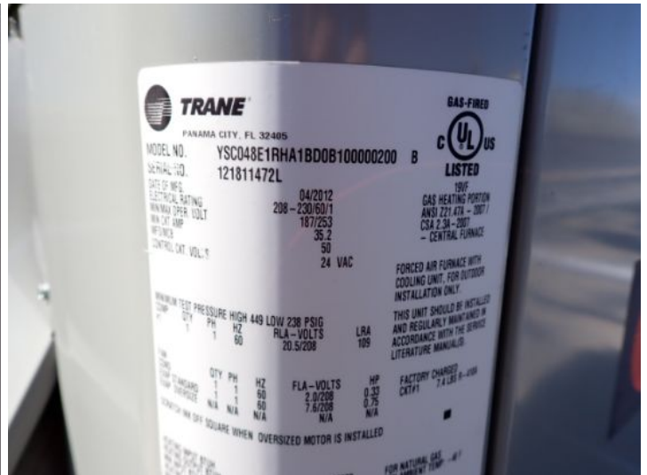
RTU 2: Trane: M/N YSC048E1RHA1BD0B100000200 B S/N 121811472L. Manufacture year 2012.
