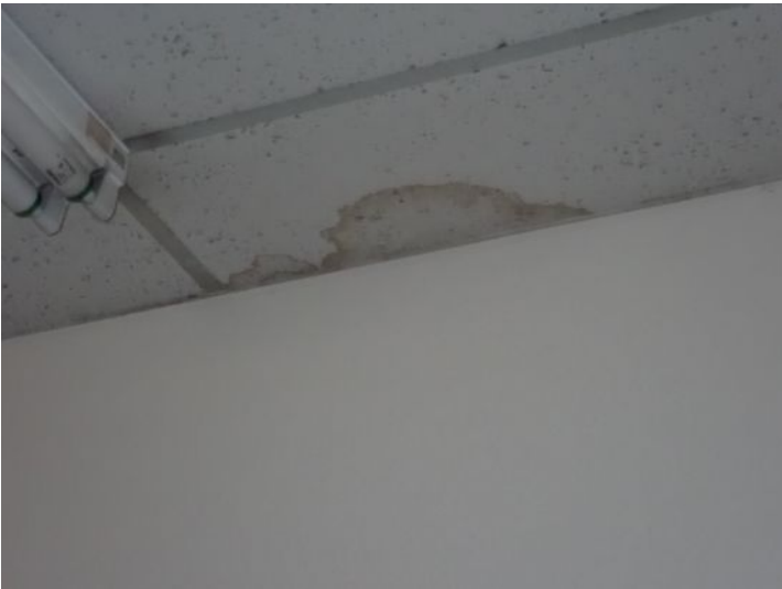
Unit 110E: Unit was vacant and will require renovations prior to placing a tenant. Recommend repairs by a licensed contractor.
