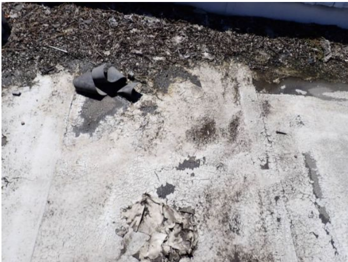
The rolled torch down roofing system above what appeared to be the old family dollar store and the vacant unit was an extremely poor condition excessive ponding feeling coding possible hail damage and excessive wear noted at the time of the inspection. Recommend complete replacement by licensed contractor.
