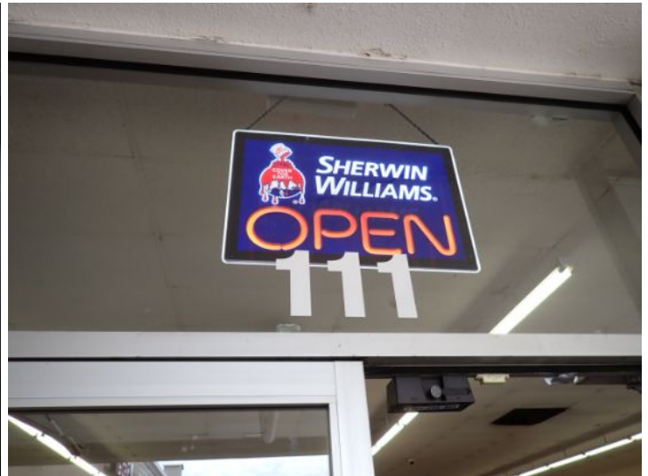
Unit 111-112: Moisture staining noted in ceiling tiles. Moisture damage noted in warehouse ceiling. Water heater not functional. Drywall ceiling damage noted. Recommend repairs.
