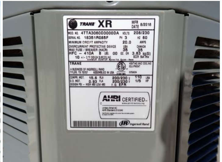
CU 4: Trane: M/N 4TTA3060D3000DA S/N 18351R085F. Manufacture year 2018.
