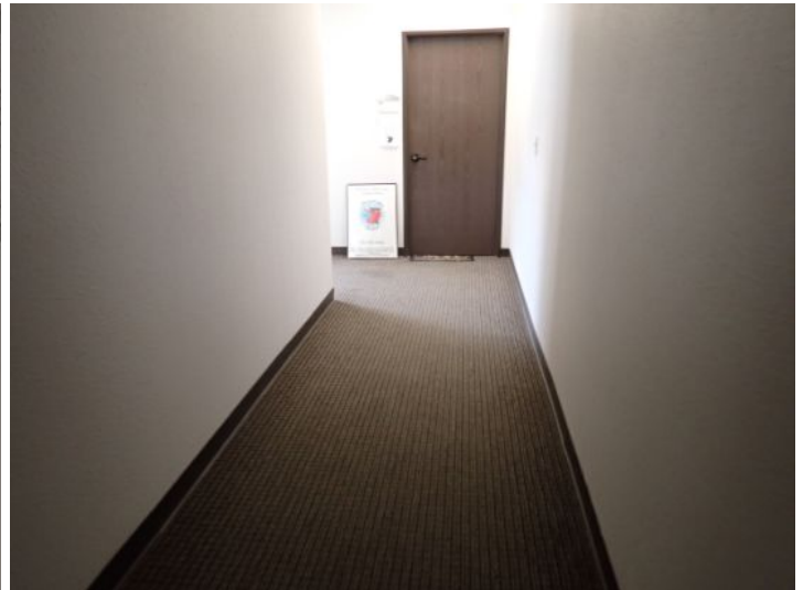
The majority of the interior common areas of the structure appeared to be in fair condition at the time of the inspection.
