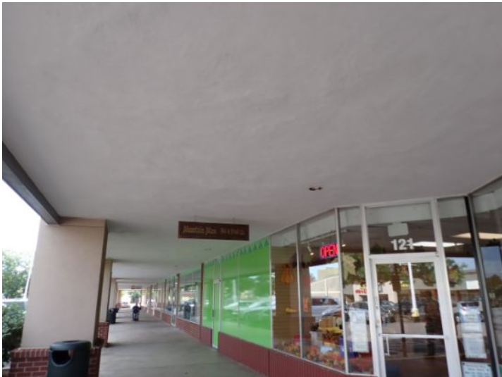
The majority of the exterior envelope of the structure appeared to be in fair condition with no significant structural movement noted at the time of the inspection.
