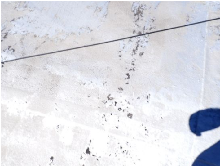
The rolled torch down roofing system above what used to be the old theater it is now currently being used as the office area appeared to be original to the structure and was showing signs of hail damage excessive ponding where and patching. Recommend replacement by licensed contractor.
