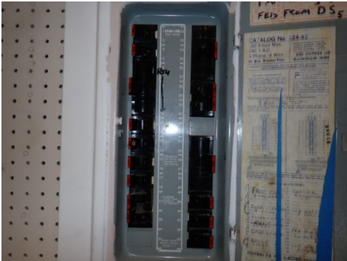
Old Federal Pacific Stab Lock breaker systems noted in some of the units at the time of the inspection. These systems have been proven to be safety/fire issues. Recommend replacement of all FPE panels and stab lock breaker systems by a licensed contractor prior to taking possession of the property.
