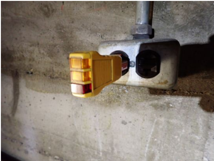
Unit 108-107: Vacant: Unit will require significant renovations prior to installing tenant. Active moisture noted in interior wall with possible microbial growth. Significant drywall damage noted in ceiling and walls in loading dock area. Basement area in poor condition. Basement bathrooms in poor condition. Electrical not working at the time of the inspection. Moisture intrusion/damage noted in basement walls. Recommend repairs as needed by a licensed contractor.
