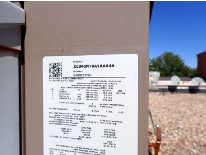
RTU 29: York: M/N ZE048N10A1AAA4A S/N N1E5737760. Manufacture year 2015.
