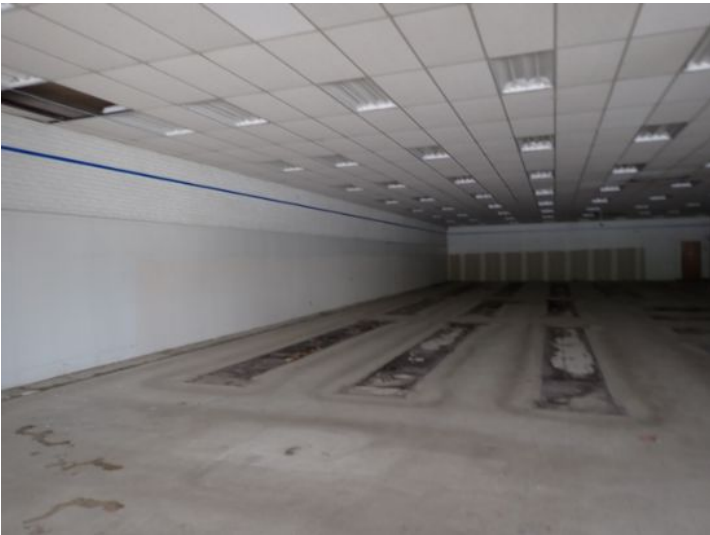
Unit 108-107: Vacant: Unit will require significant renovations prior to installing tenant. Active moisture noted in interior wall with possible microbial growth. Significant drywall damage noted in ceiling in loading dock area. Basement area in poor condition. Basement bathrooms in poor condition. Electrical not working at the time of the inspection. Moisture intrusion/damage noted in basement walls. Recommend repairs as needed by a licensed contractor.
