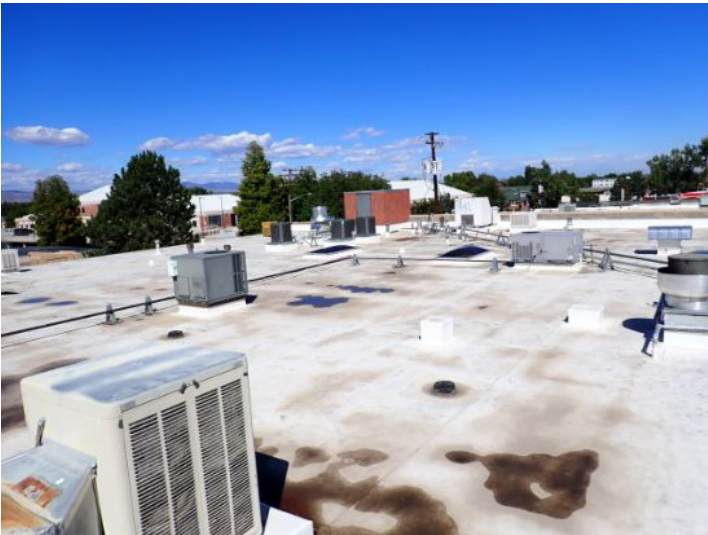
TPO roofing membrane located above the mall area of the property while appearing to be in fair condition was showing signs of excessive deferred maintenance and ponding at the time of the inspection. Recommend repairs by licensed contractor.
