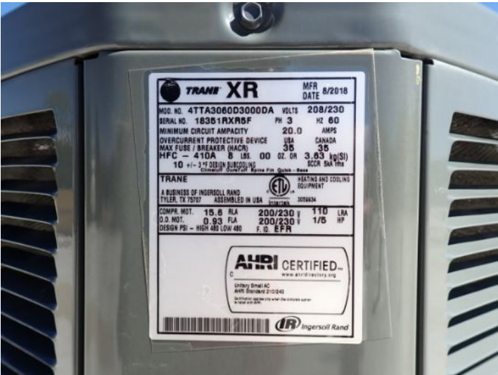
CU 3: Trane: M/N 4TTA3060D3000DA S/N 18351RXR5F. Manufacture year 2018.
