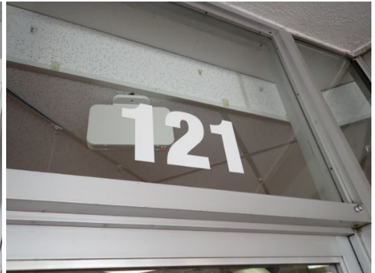
Unit 121: VCT flooring damage noted. Recommend repairs.
