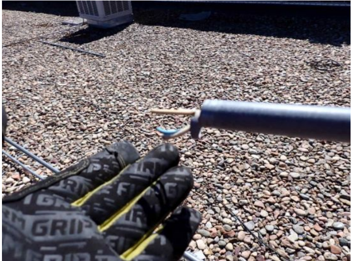
Exposed electrical wiring noted in areas around the exterior and on the roof of the structure at the time of the inspection. Recommend proper repairs by a licensed electrician.
