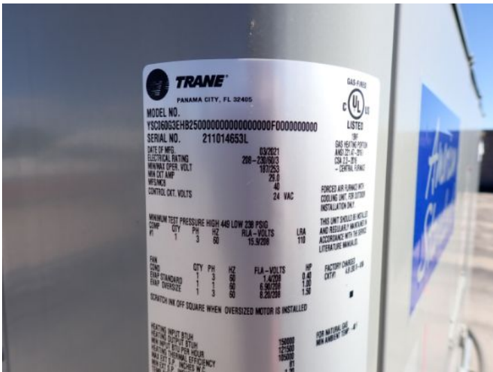
RTU 21: American Standard: M/N YSC060G3EHB25000000 S/N 211014653L. Manufacture year 2021.
