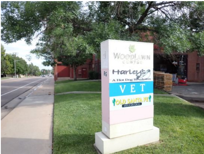
Signage appeared to be in fair condition at the time of the inspection.
