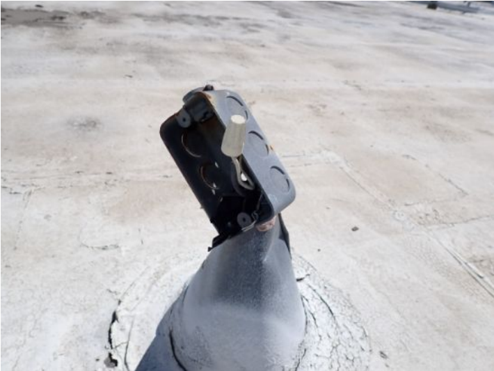
Exposed electrical wiring noted in areas around the exterior and on the roof of the structure at the time of the inspection. Recommend proper repairs by a licensed electrician.
