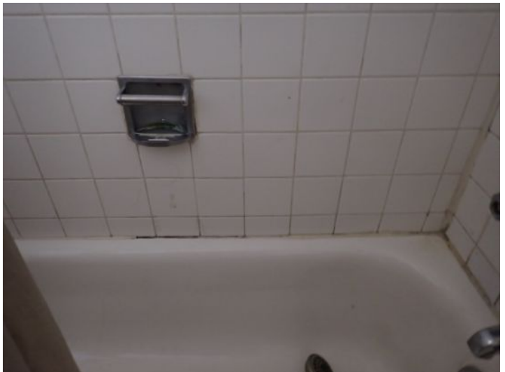
Unit 22: Carpeting in poor condition. Vinyl flooring damage noted. Missing dead cover on electrical panel. Wall damage noted in bathroom. Cracked mirror on closet door. Recommend repairs.
