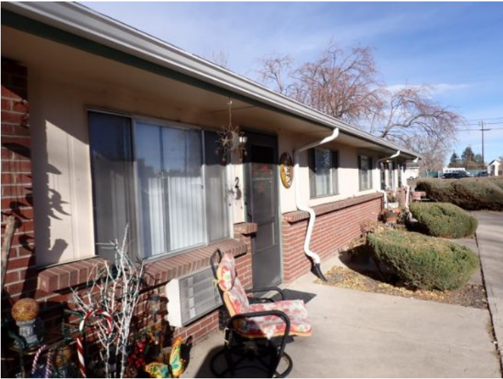
The majority of the exterior envelopes of the structures appeared to be in fair condition at the time of the inspection.
