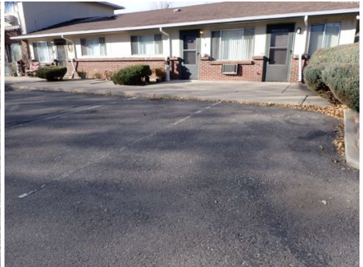
The parking lot surface was in fair condition at the time of the inspection.
