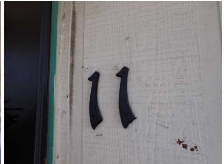
Unit 11: Front door trim damaged. Significant flooring deflection. Flooring damage noted. Recommend repairs.
