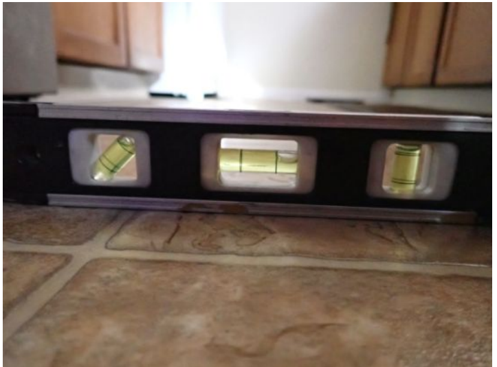
Unit 18: Carpet damage noted. Tub/shower surround requires caulk/grout repairs. Significant flooring deflection noted. Recommend repairs.
