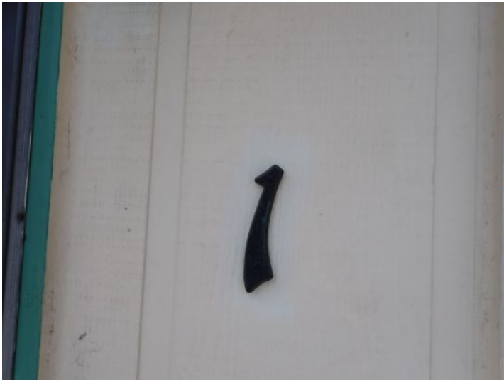
Unit 1: Significant floor deflection noted. Missing bedroom door. Significant wall/ceiling junction cracking noted. Carpet damage. Significant floor settling noted. Recommend repairs.
