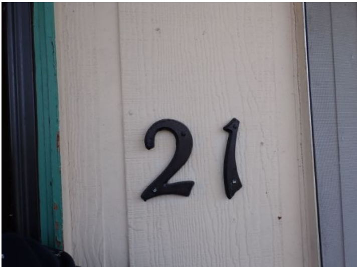
Unit 21: Missing cover plate noted on electrical panel. Wall damage noted in bathroom. Flooring damage noted. Tub spigot missing. Recommend repairs.
