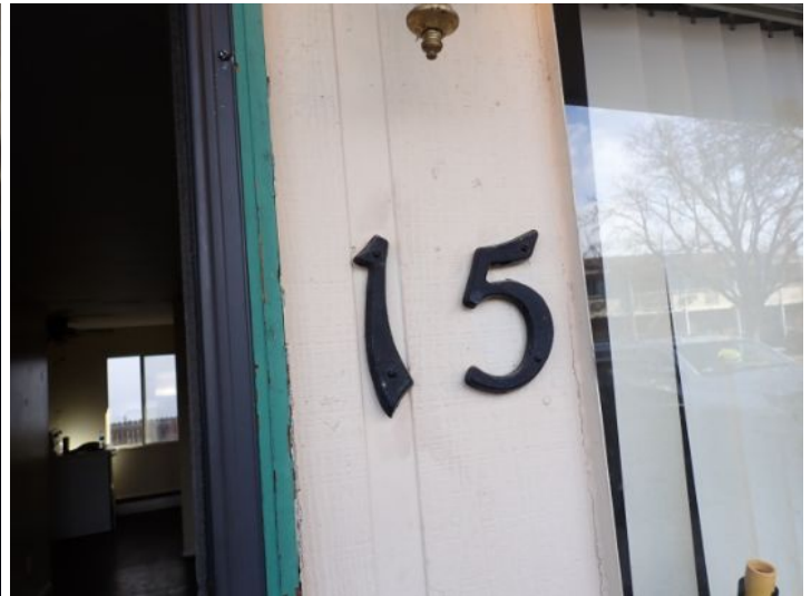
Unit 15: Unit being turned at the time of the inspection.
