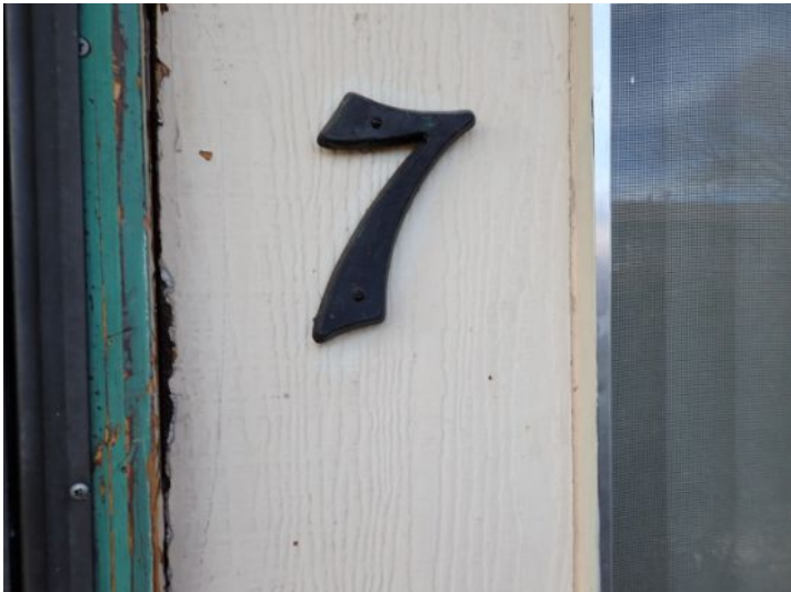
Unit 7: No significant findings noted at the time of the inspection.
