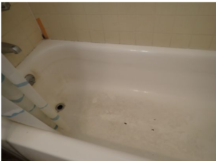
Unit 9: Ceiling cracking. Sub standard plumbing noted below kitchen sink. Carpet in poor condition. Tub finish in poor condition. Recommend repairs.
