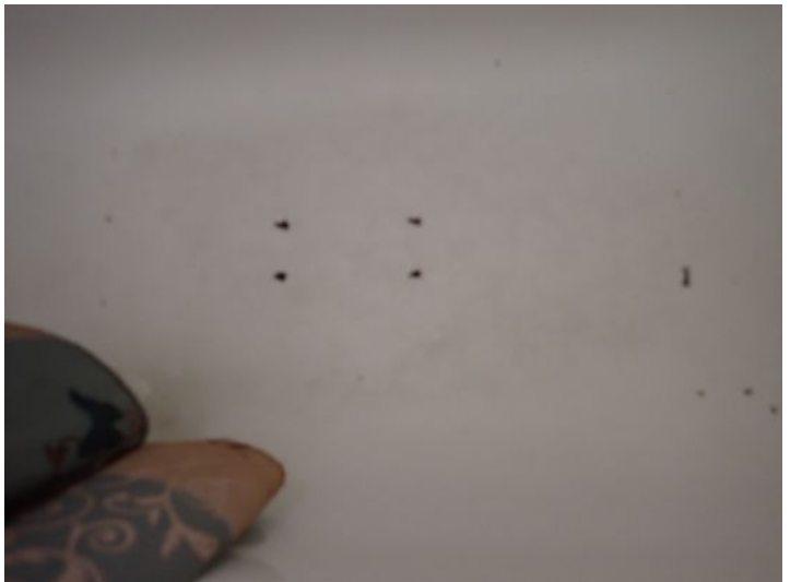
Unit 10: Flooring damage. Tub/shower surround requires caulk/grout repairs. Tub finish in poor condition. Broken bathroom window glass. Recommend repairs.
