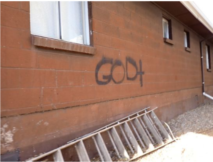
The majority of the exterior envelopes of the structures appeared to be in fair condition at the time of the inspection.
