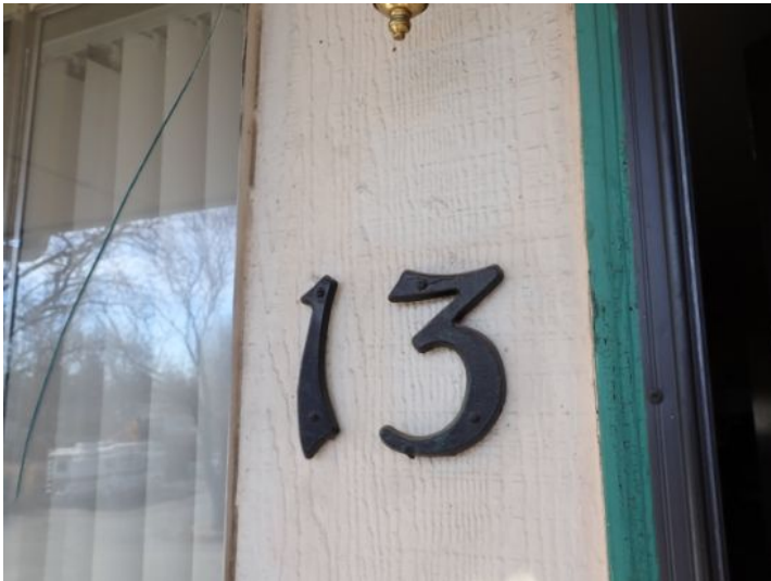
Unit 13: Cracked window glass. Broken window glass in rear of unit. Tub/shower surround requires caulk/grout repairs. Tub finish in poor condition. Closet door damage noted. Vinyl flooring damage noted. Recommend repairs.
