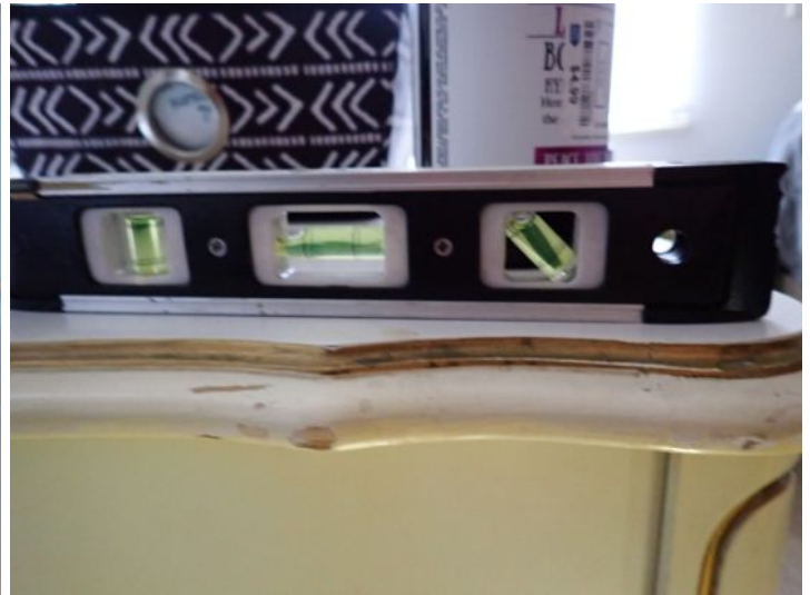
Unit 1: Significant floor deflection noted. Missing bedroom door. Significant wall/ceiling junction cracking noted. Carpet damage. Significant floor settling noted. Recommend repairs.
