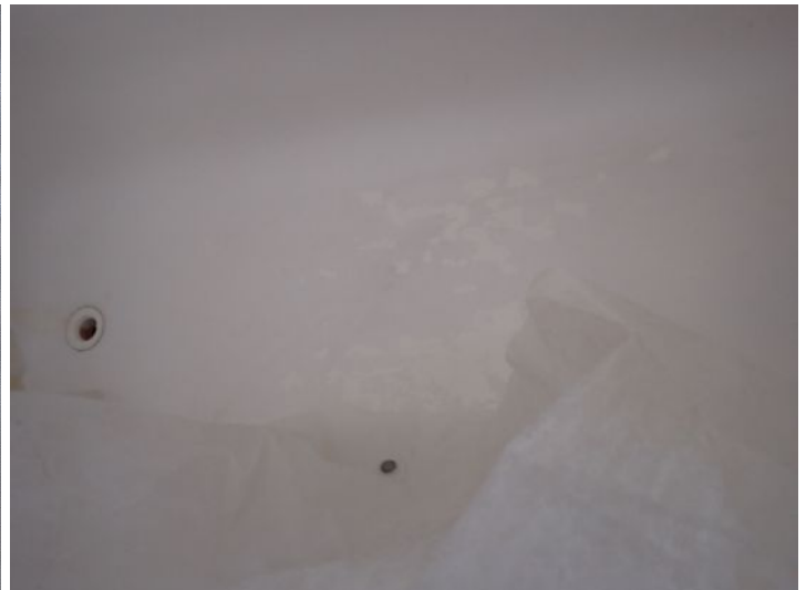
Unit 5: Tub finish in poor condition. Recommend repairs.
