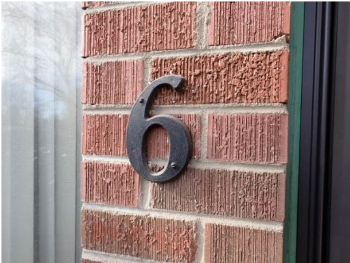
Unit 6: Kitchen sink faucet leaking at valve handle. Recommend repairs.
