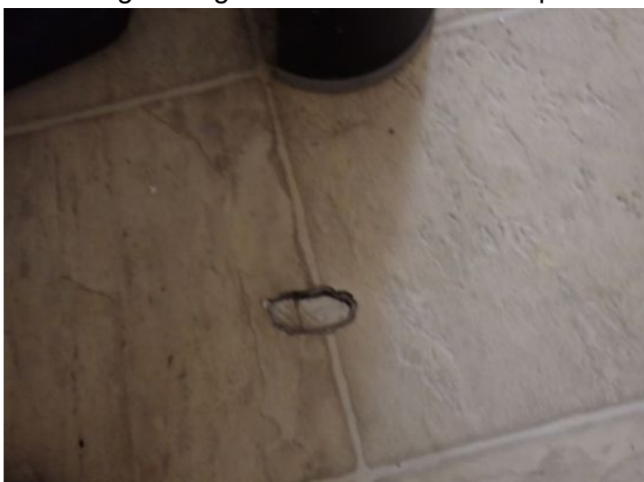
Unit 13: Cracked window glass. Broken window glass in rear of unit. Tub/shower surround requires caulk/grout repairs. Tub finish in poor condition. Closet door damage noted. Vinyl flooring damage noted. Recommend repairs.
