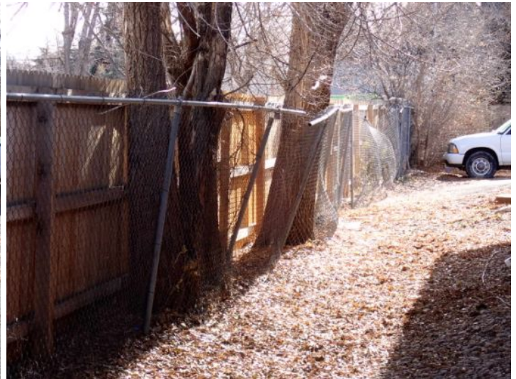
Fencing damage noted around the property at the time of the inspection. Recommend repairs by a licensed contractor.
