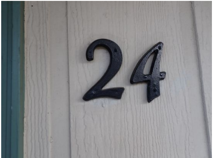
Unit 24: Carpet in poor condition. Ceiling/wall junction cracking. Vinyl floor damage. Wall damage noted below kitchen sink. Recommend repairs.
