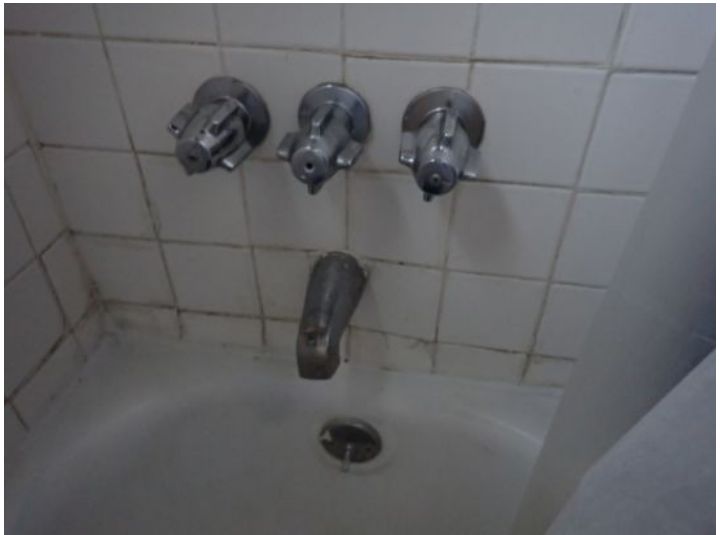
Unit 18: Carpet damage noted. Tub/shower surround requires caulk/grout repairs. Significant flooring deflection noted. Recommend repairs.
