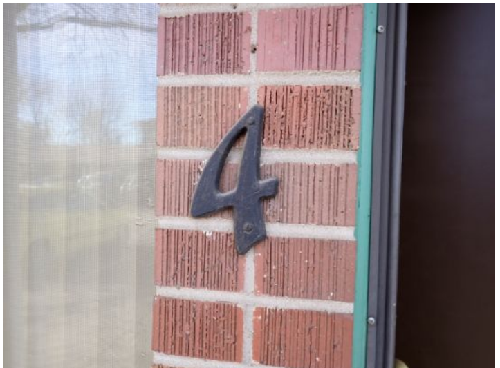
Unit 4: Kitchen counter and wall separation noted. Vanity sink rusting. Past moisture damage noted in bathroom wall but no moisture present at the time of the inspection. Recommend repairs.
