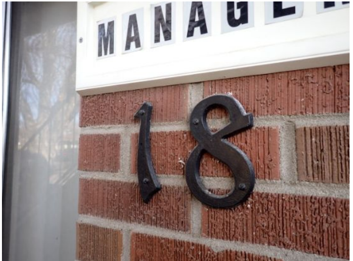
Unit 18: Carpet damage noted. Tub/shower surround requires caulk/grout repairs. Significant flooring deflection noted. Recommend repairs.
