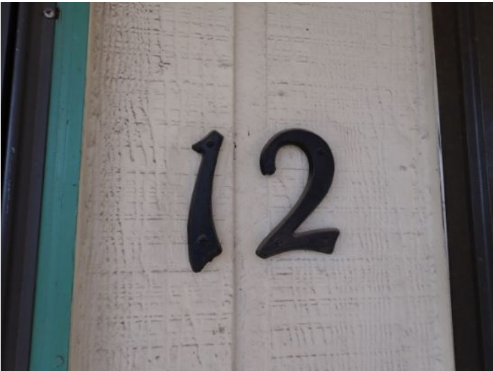
Unit 12: Carpet in poor condition. Vinyl flooring damage. Moisture damage noted below bedroom window. Recommend repairs.
