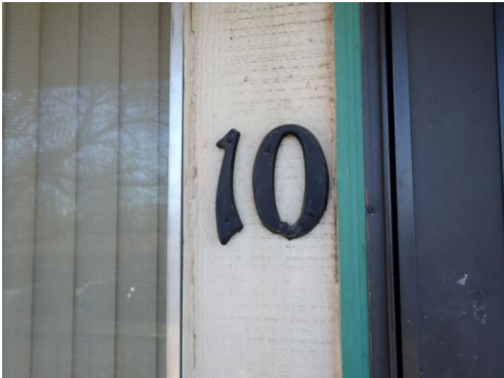
Unit 10: Flooring damage. Tub/shower surround requires caulk/grout repairs. Tub finish in poor condition. Broken bathroom window glass. Recommend repairs.
