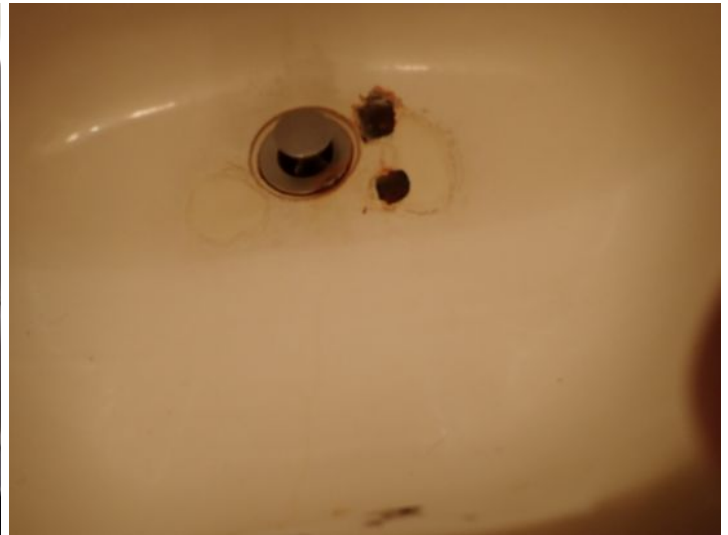
Unit 4: Kitchen counter and wall separation noted. Vanity sink rusting. Past moisture damage noted in bathroom wall but no moisture present at the time of the inspection. Recommend repairs.
