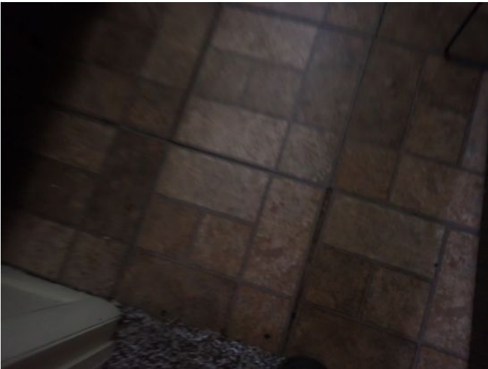
Unit 24: Carpet in poor condition. Ceiling/wall junction cracking. Vinyl floor damage. Wall damage noted below kitchen sink. Recommend repairs.
