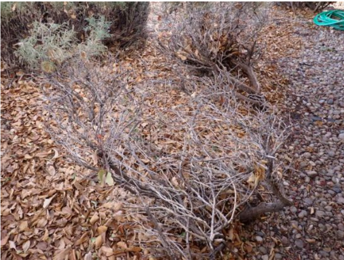
Foliage in contact with structure at time of inspection. Recommend trimming/removal.
