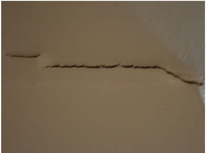
Unit 2: Tub/shower surround requires caulk/grout repairs. Significant ceiling cracking noted. Significant wall movement noted. Recommend repairs.
