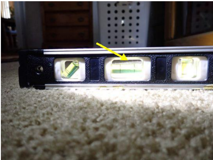
Unit 1: Significant floor deflection noted. Missing bedroom door. Significant wall/ceiling junction cracking noted. Carpet damage. Significant floor settling noted. Recommend repairs.
