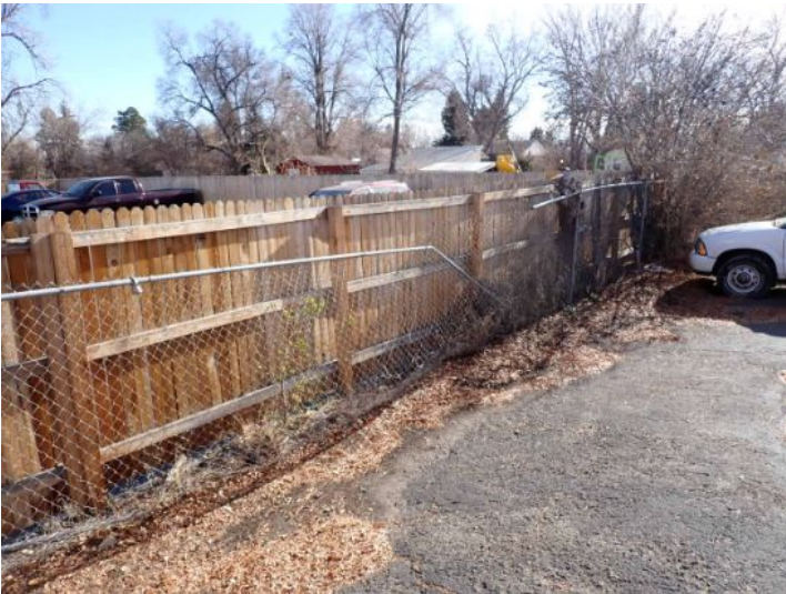
Fencing damage noted around the property at the time of the inspection. Recommend repairs by a licensed contractor.
