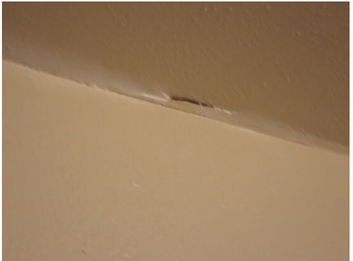
Unit 20: Damaged radiator system noted. Significant flooring deflection noted. Tub finish in poor condition. Significant wall movement noted. Recommend repairs.
