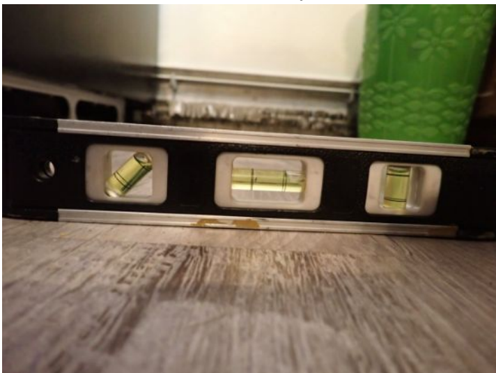
Unit 20: Damaged radiator system noted. Significant flooring deflection noted. Tub finish in poor condition. Significant wall movement noted. Recommend repairs.
