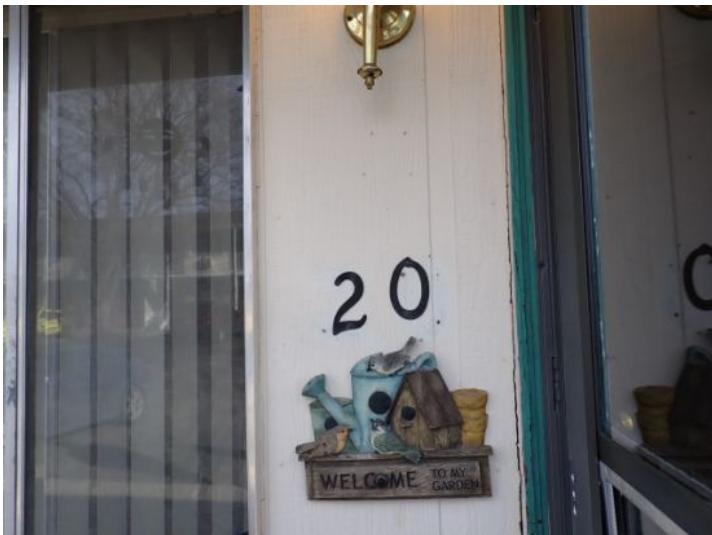
Unit 20: Damaged radiator system noted. Significant flooring deflection noted. Tub finish in poor condition. Significant wall movement noted. Recommend repairs.
