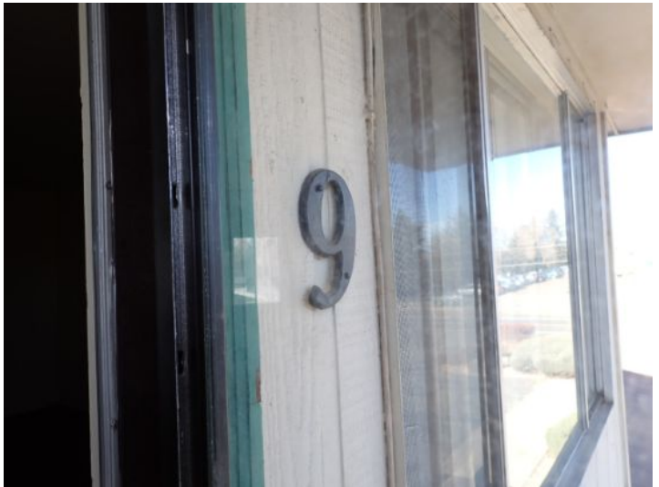
Unit 9: Ceiling cracking. Sub standard plumbing noted below kitchen sink. Carpet in poor condition. Tub finish in poor condition. Recommend repairs.
