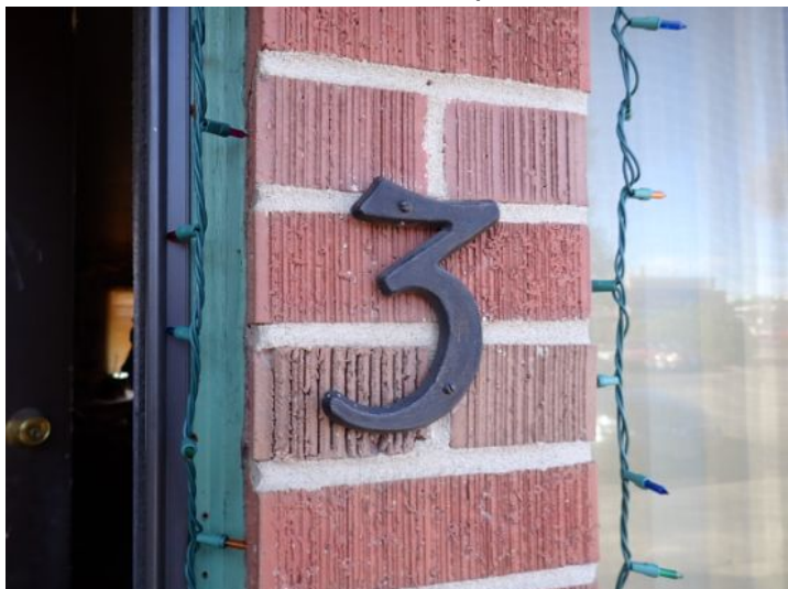
Unit 3: Carpet damage. Separation noted between kitchen counter and wall. Kitchen cabinet failure noted. Vinyl flooring damage. Tub/shower surround requires caulk/grout repairs. Bedroom closet door damage noted. Recommend repairs.
