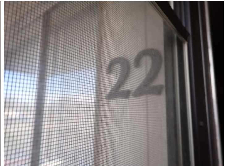
Unit 22: Carpeting in poor condition. Vinyl flooring damage noted. Missing dead cover on electrical panel. Wall damage noted in bathroom. Cracked mirror on closet door. Recommend repairs.
